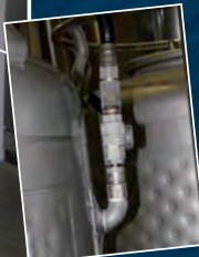
Stainless steel quick coupling system (drip and run free)
